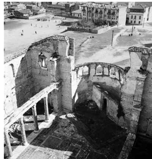
[7] Picture by Nicholas V. Artamonoff in 1937: a view from the minaret with an oblique wall and platform in the former apse revealing the second life of the Stoudios Monastery church as a mosque.
