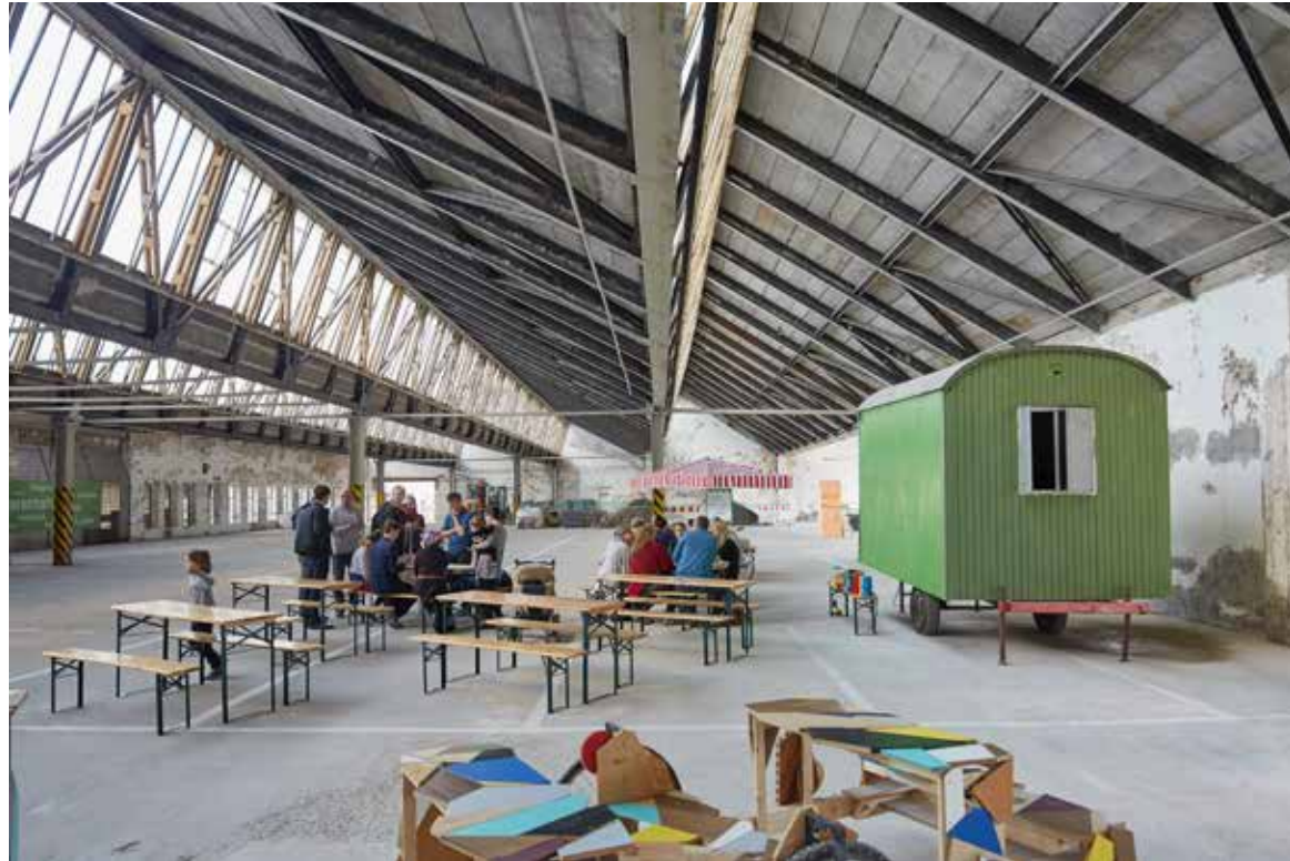
[2] The interior of the shed hall of the Samtweberei in Krefeld.
