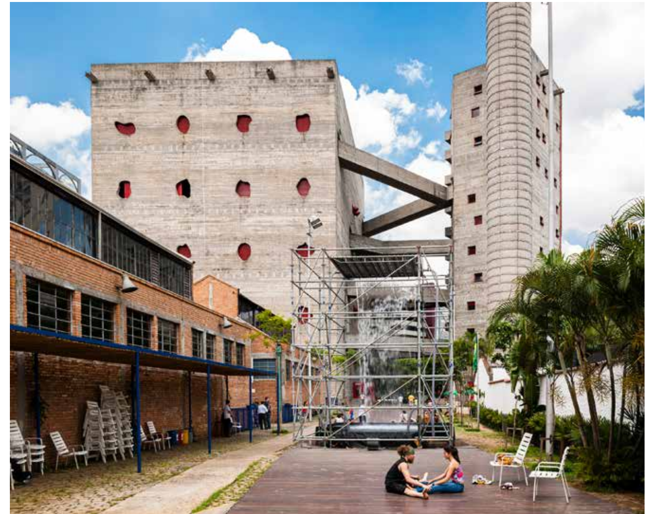
[1] The wooden link between old and new architecture at the SESC Pompeia cultural centre in São Paulo, Brazil.
