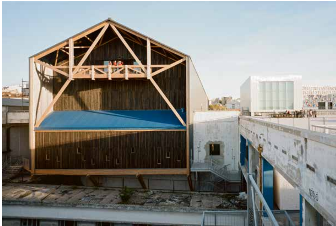
[4] La Friche went through several transformation processes to gradually adapt to the multiple needs of its users.
