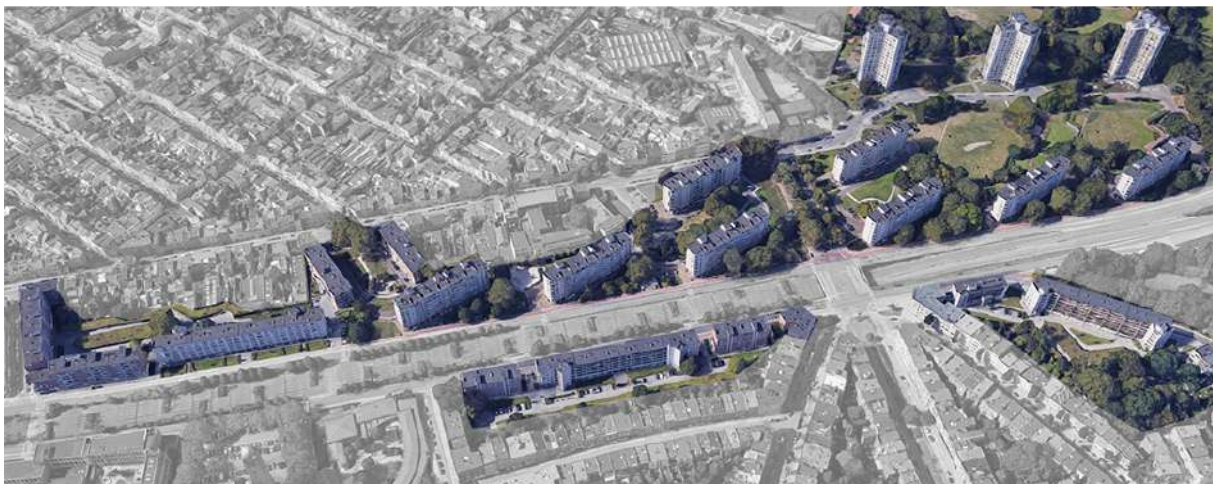
Fig. 1 – Areal view of the Jan De Voslei in Antwerp. Source: Google Earth, edited by Marie Moors.
