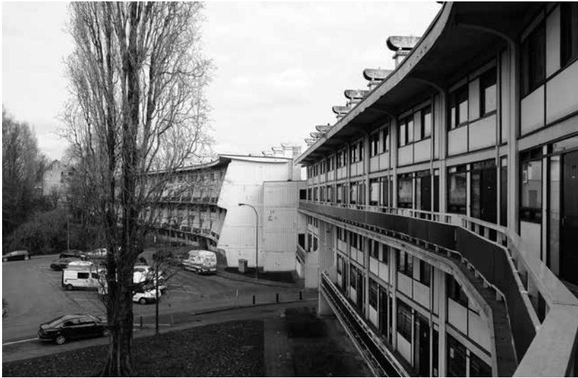
PHOTOGRAPH OF THE SOUTHERN RESIDENTIAL BLOCKS WITH VIEW TOWARD THE GALLERY LEADING TO TWO-STOREY APARTMENTS, ARENAWIJK ANTWERP (BE), 2021
