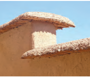
top of a wall made of adobe and reed
