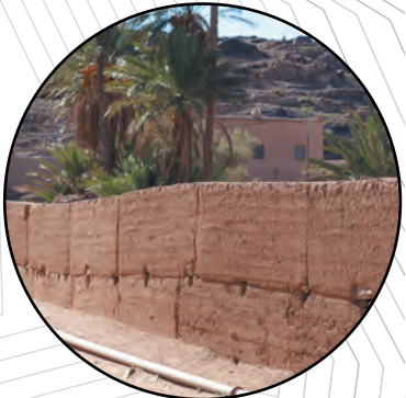
Even with only a few rainy days per year, rammed earth walls need to be detailed well to be protected against water damage
