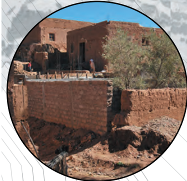
Building with both rammed earth (right) and concrete blocks (left)
