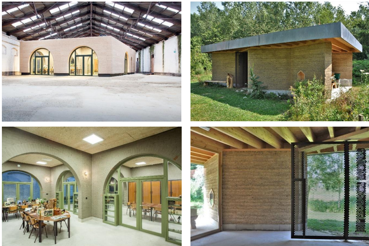
Figure 2. Left: Load-bearing CEB-walls with exterior hempcrete insulation in the Bio Class (©Thomas Noceto). Right: Naked load-bearing rammed earth walls in the Bee Hall (©Ken Dupont).
