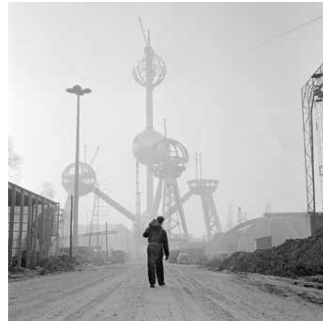
[2] The Atomium under construction, Brussels Expo 58. © Dolf Kruger / Nederlands Fotomuseum
