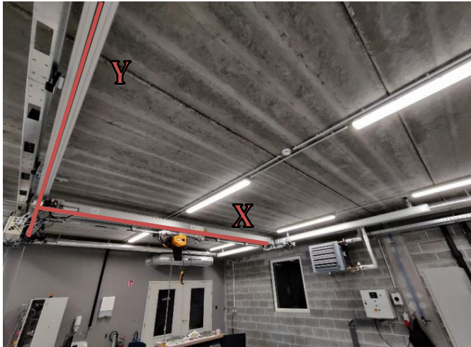
Figure 9: a dual axis overhead crane to test the Follow-Me principle.
