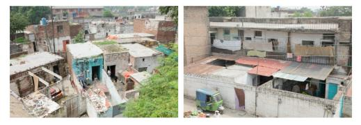
**Figure 2.** Pacca houses with brick-made structure (**left**); Katcha structure using galvanized sheets (**right**) representing buildings' typology in Hope Colony. (Source: Photos taken by the first author).
