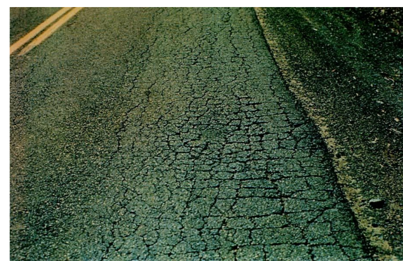
Figure 2: Alligator or bottom-up cracking [2]
