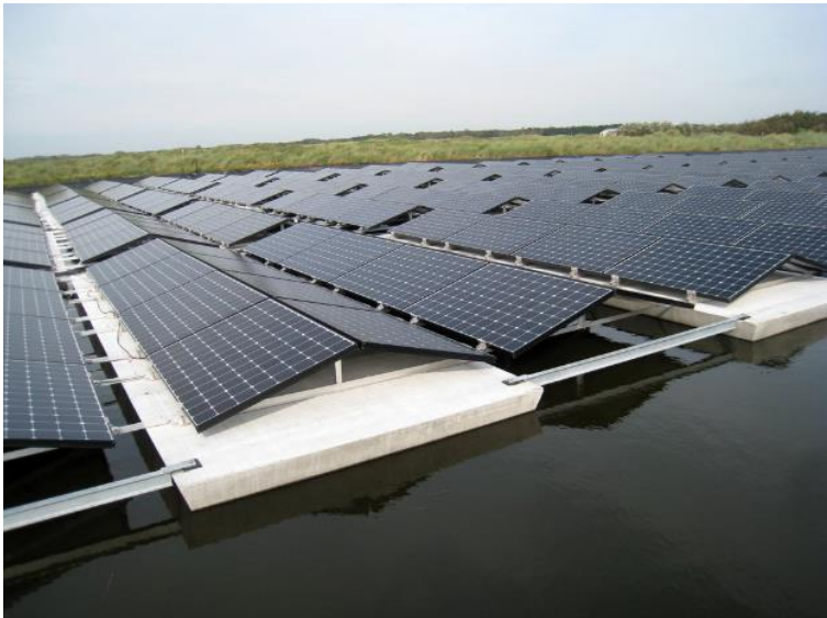
Figure 13: Modules in gable configuration [39]
