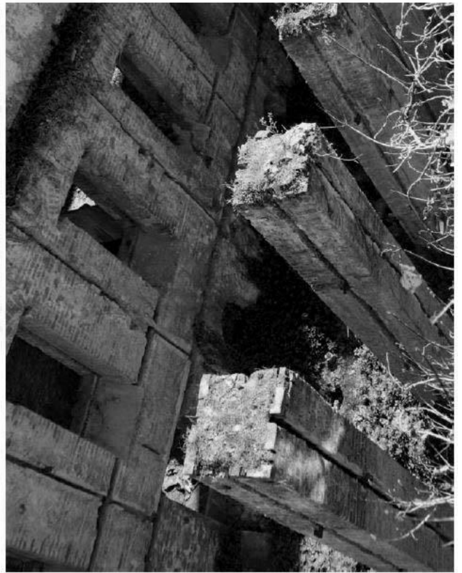
Figure 26 - Current situation of the columns of the warehouse
