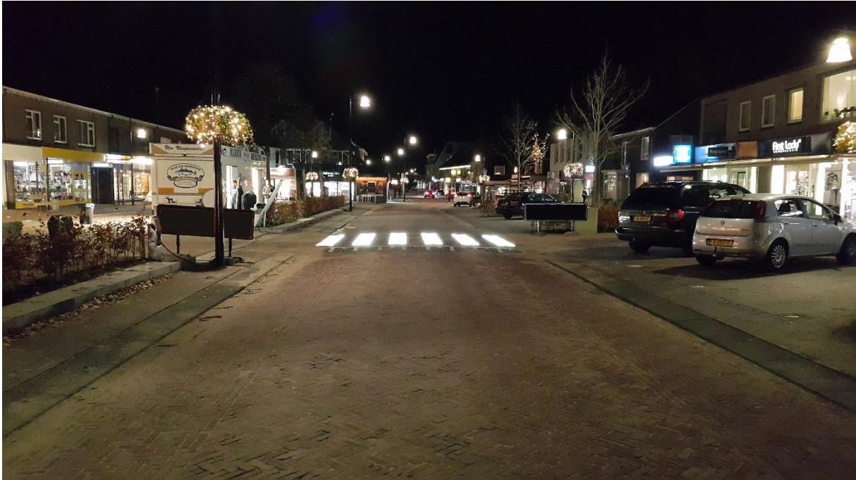
Figuur 6: Lighted Zebra Crossing (Lighted Zebra Crossing B.V., z.d.b)
