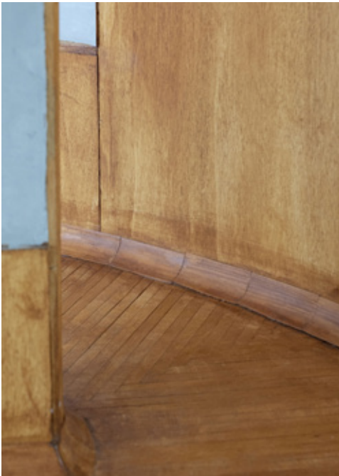
Fig. 11.4 MDF and veneer model of a passage in the original museum, scale 1:5, Shamila Gostelow and Silja Siikki, detail. Photograph: Bas Leemans.
