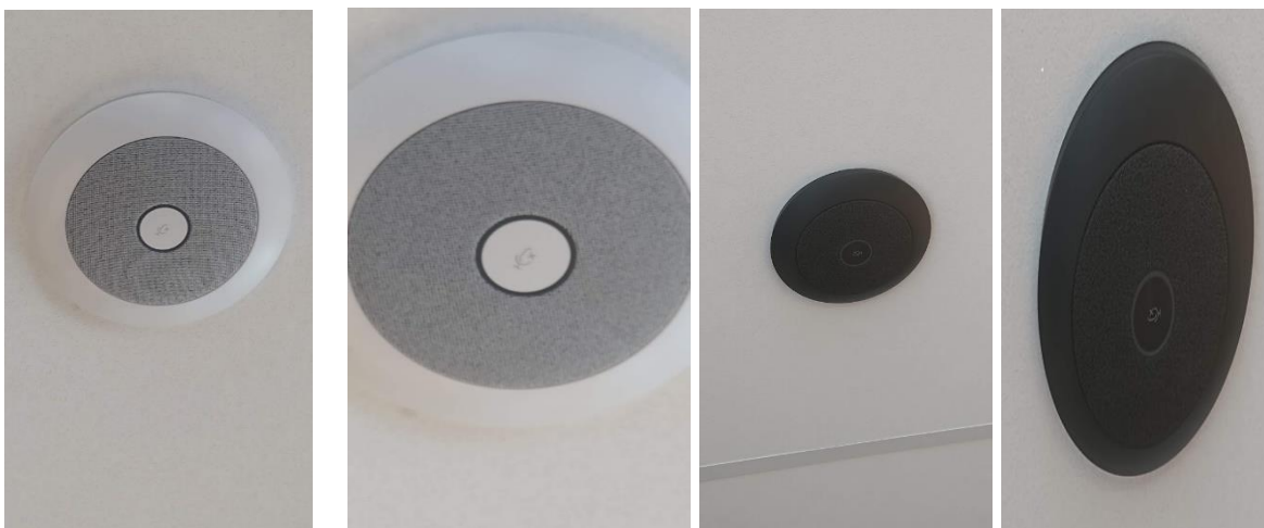
Image 1: Example of speakers attached to the ceiling in-office rooms for hybrid work
