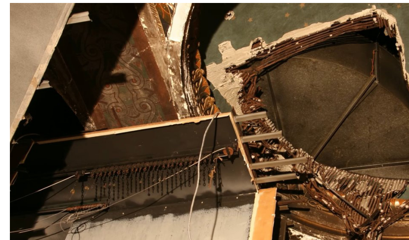
Figure 18: Photo of cupola pierced with ventilation system. Danielle Demers (2015).
