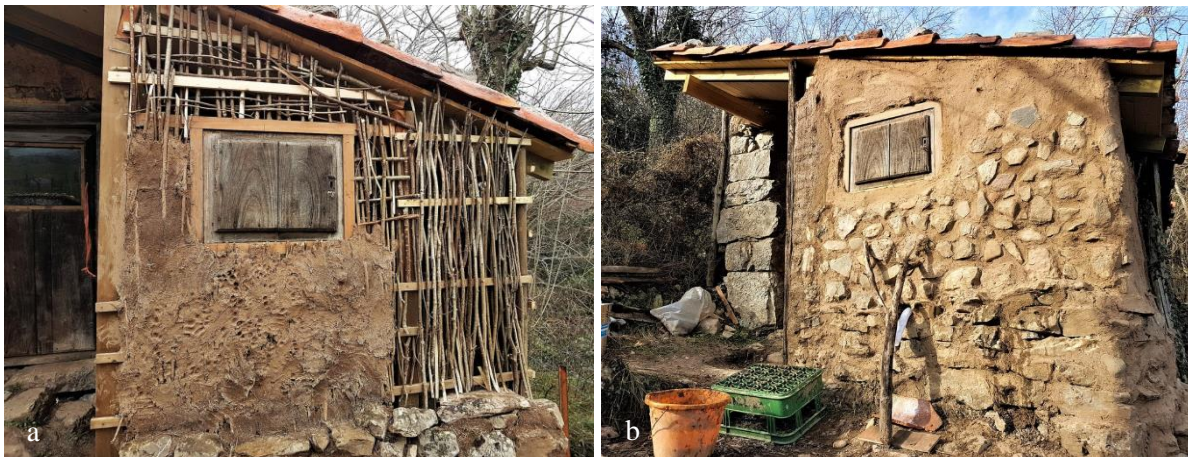
Figuur 6: Toepassing wattle and daub [14]
