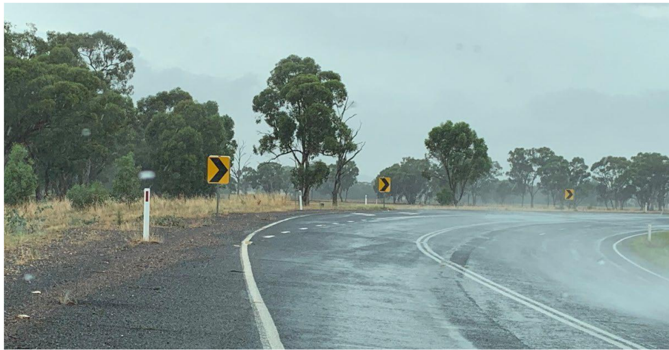
b) Example of seal joint that could confuse MV
