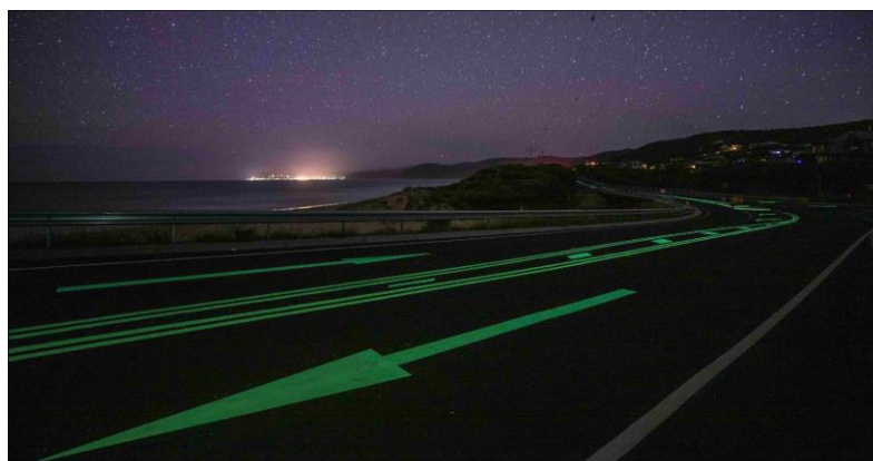
Figure 6 Luminescent road markings applied in Australia (Source: [40])
