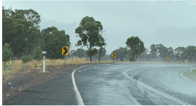
b) Example of seal joint that could confuse MV
