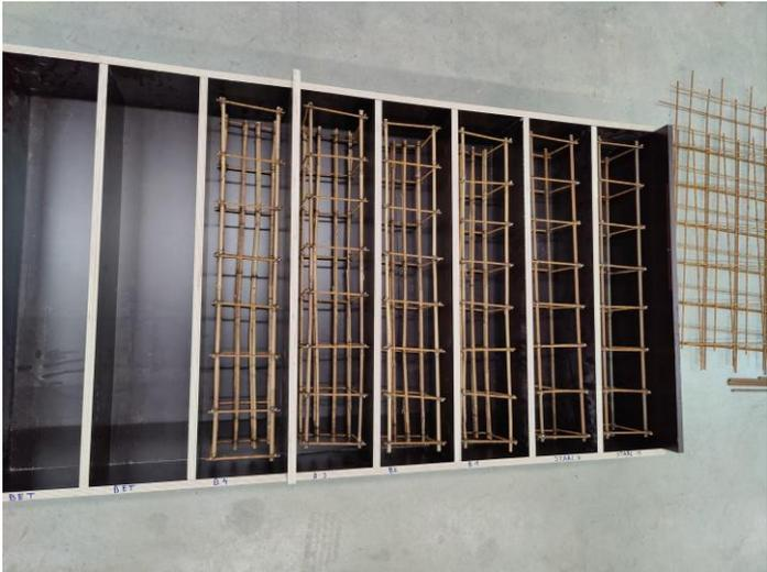
Figure 24: Formwork for the small beams
