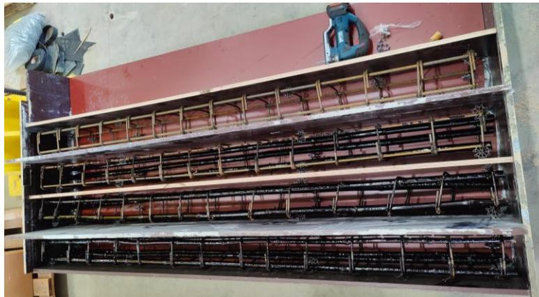
*Figure 32: Formwork for the large beams*
