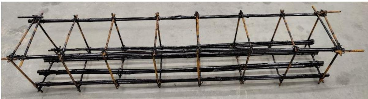
*Figure 23: Reinforcement cage for BBRC*
