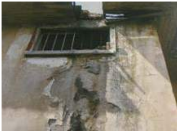
Figure 33 The demolished facade on the eastern facade. (Kalan Mühendislik, 2008)
