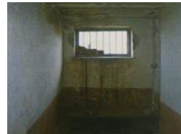
Figure 29 This view is right before turning to the hallway in fig. 26. (Kalan Mühendislik, 2008)
