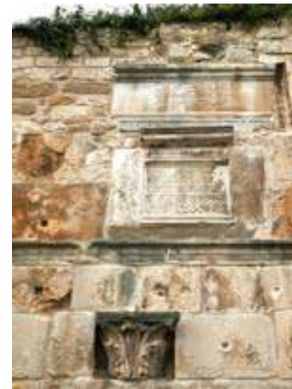
Figure 8 An obvious example. Different regimes reused architectural pieces to rebuilt the walls by showing their victory.
