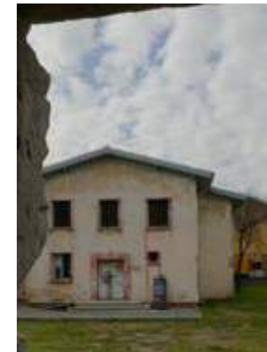
Figure 24 The corners of the building with the isolation cells and the facade is an example of the detachment.
