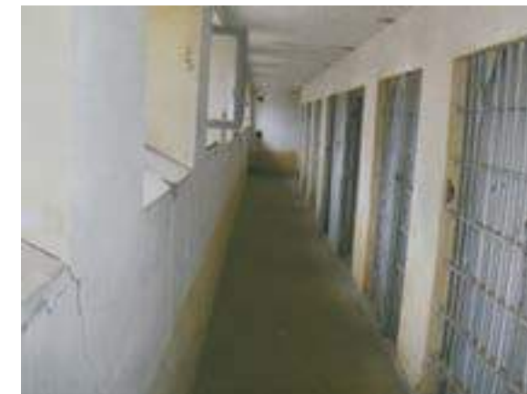
Figure 27 The hallway in front of the cells of the southern facade. (Kalan Mühendislik, 2008)
