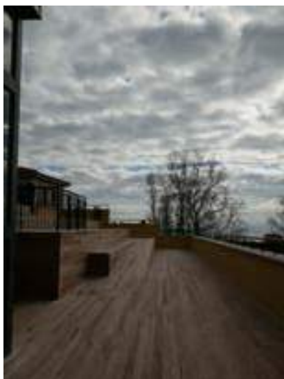
Figure 20 This is the viewpoint built after the renovation of 2023, it represents the guardposts. and is on top of the building in fig. 21.
