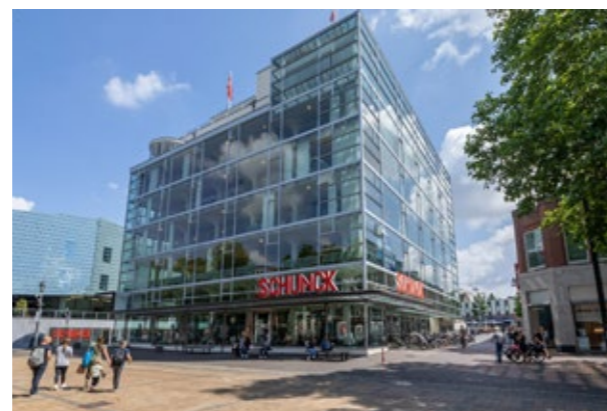
Fig. 3.23 The Schunck building now, retrieved from www.heerlenmijnstad.nl in 2023.
