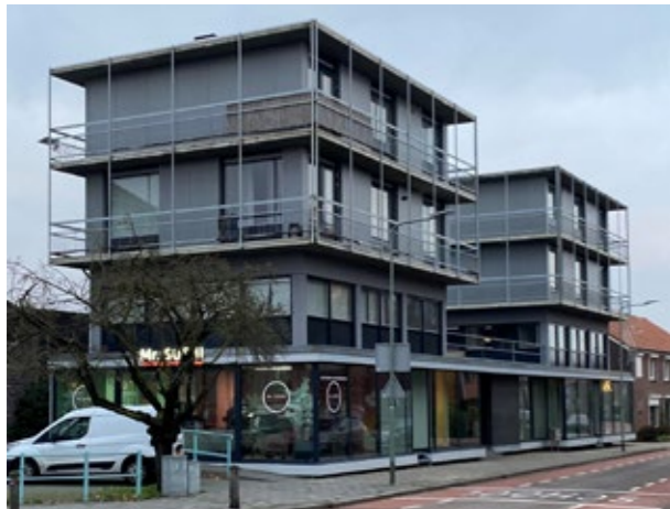
Fig. 3.33 Pand Mooren in the current state, picture dated 17-12-2022.
