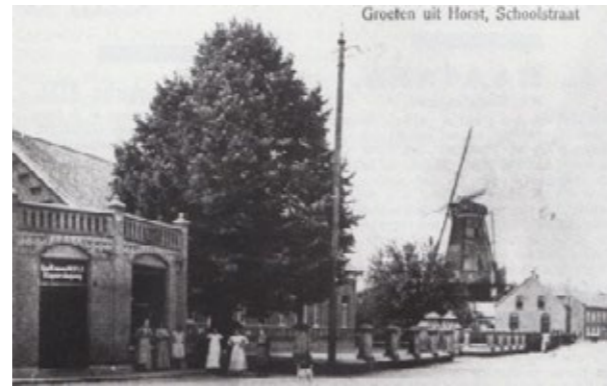
3.8.1 View across of the street of the location where Pand Mooren would later be built. Beuijsse meule in the background. Dated about 1920
