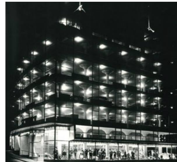
Fig. 3.24 The Schunck building by night in 1935, made by J. Cohnen retrieved from the book Schunck's Glass Palace of 2016 .
