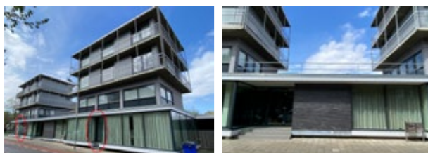
Fig. 4.4 Pand Mooren in the current state, the front façade. On the left the two new entrances to the towers are indicated with red circles and on the right the middle part of the façade in black bricks. Own pictures, dated 25-4-2023.
