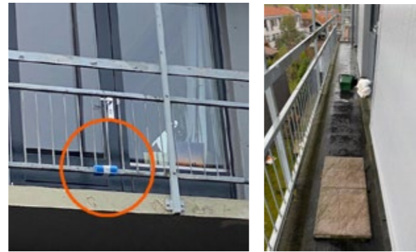
Fig. 4.5 Detail of the foam protection around the railings in Pand Mooren and the limited space in the galleries, Own pictures, dated 16-02-2023 and 25-04-2023.
