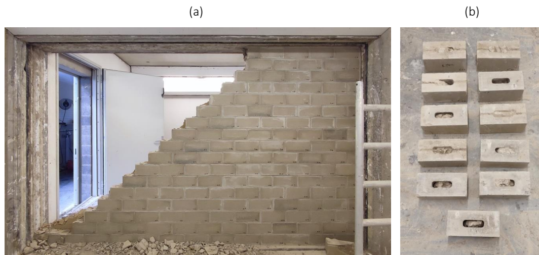
Figure 4. Deconstruction of prototype wall (a) and compressed earth blocks after cleaning (b).
