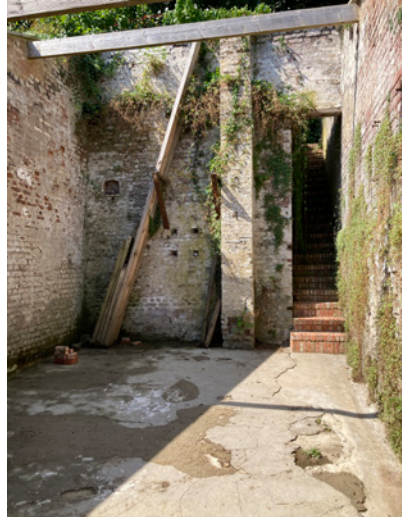
Fig. 10: New exterior courtyard created by removing the dilapidated roof of the former stable. Photograph by the author.
