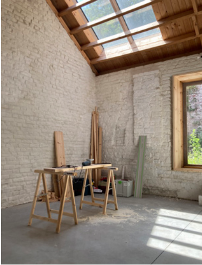
Fig. 9: Interior of the former gunsmith's atelier during renovation into a maisonette. Photograph by the author.
