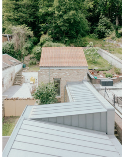
Fig. 14: The same view of the newly reconstructed and extended annexe, showing the roof spanning from party wall to party wall. Photograph by Jeremy Piret. Courtesy of Simon Pirlot Architecte.
