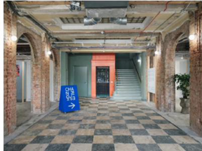
Fig. 4: Same view of the entrance hall after the recent renovation. Photograph by Henry Woide. Courtesy of Material Cultures.
