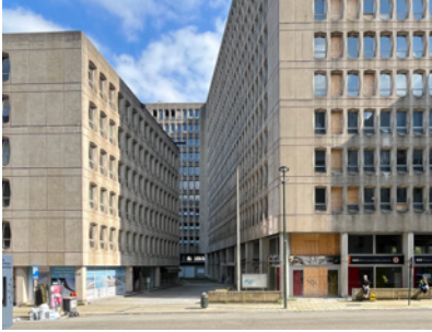
Fig. 15: Current exterior view of the former SECO building, part of an ensemble situated between Rue d'Arlon/Aarlenstraat and Trierstraat/Rue de Trèves in the European Quarter of Brussels. Photograph by the author.
