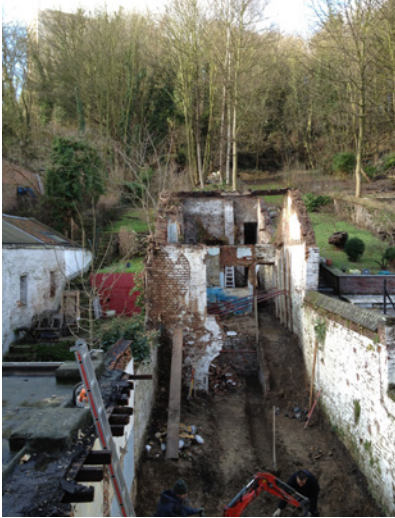
Fig. 13: View of the annexe during construction, showing the excavation of the future living space between the two party walls. Photo courtesy of Simon Pirlot Architecte.
