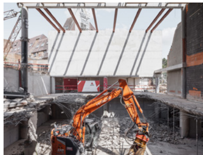
Fig. 21: Cutting through the dalle below Louvain-la-Neuve to excavate the new space for Atelier Théâtre Jean Vilar. Photograph by Corentin Haubruge. Courtesy of Ouest architecture.
