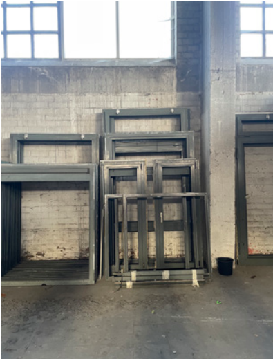
Impact Factory project: Steel window frames being reclaimed from a nearby demolition site in Mechelen. Storage of the window frames and design exercise for positioning of the reclaimed frames in the front façade, WIT architecten
