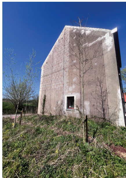
Figure 81. Photograph of one of the buildings at the Ferme du Chaudron project, Brussels, April 2025. Photo by the author.
