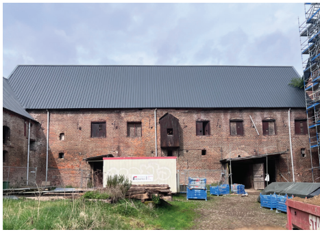
Figure 107. Current state of stables - housing intervention zone. Frontal facade from courtyard.
