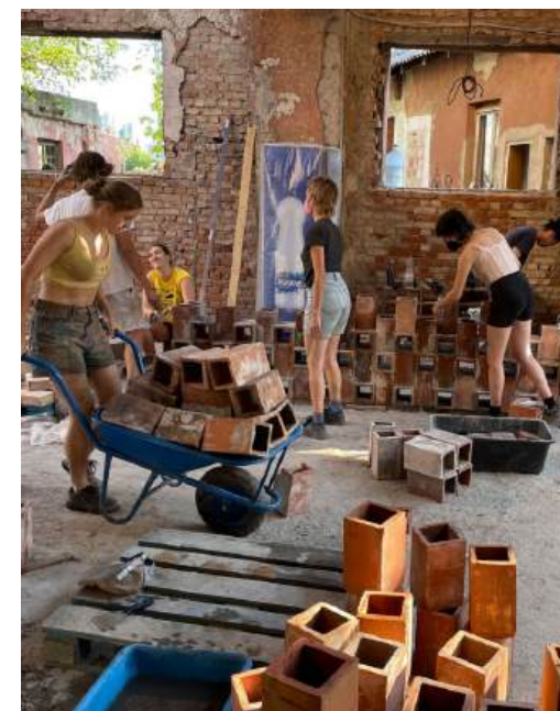
Figure 4.17 Bar construction of reclaimed bricks found on site.
