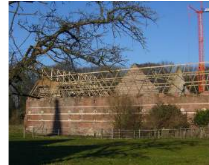
Figure 1.12 New roof construction of the farm building for the installation of emergency roofs.
