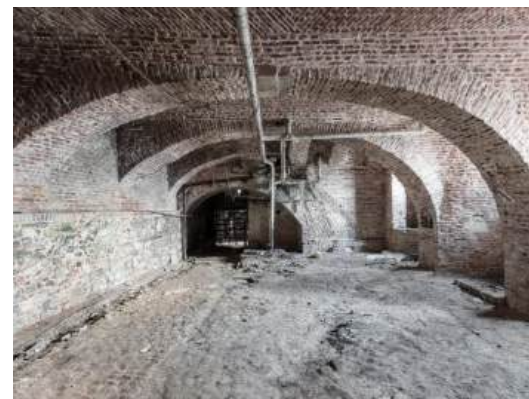
Figure 1.19 Vaulted ceiling structure of the basement in the castle.
