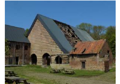
Figure 1.14 Installation of emergency roof on the tithe barn.
