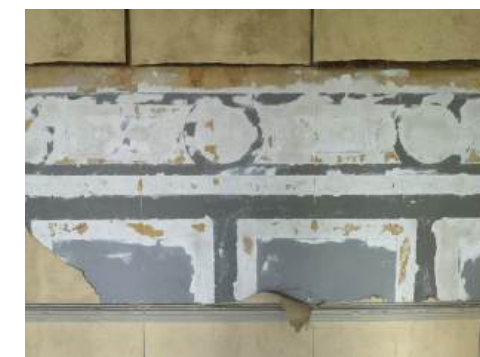
Figure 3.16 Different historical wall layers exposed.
