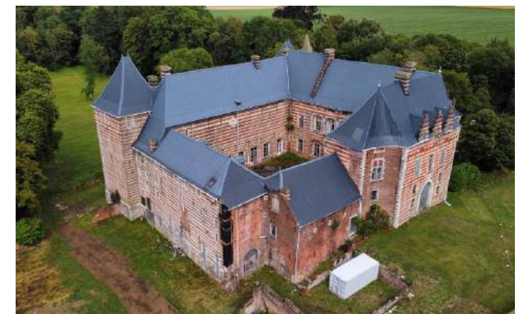
Figure 1.4 Enclosed west and south facades.
