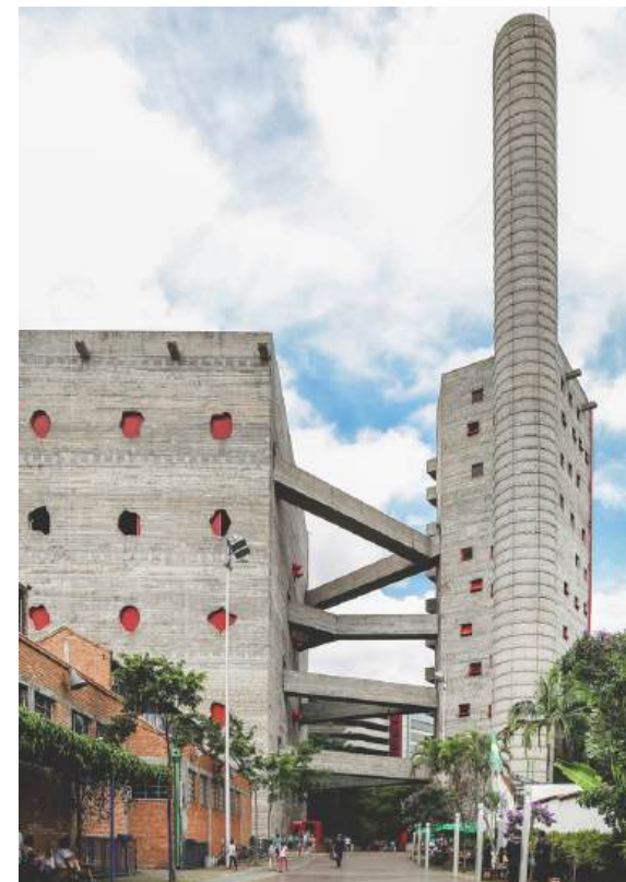
Figure 4.5 Three new concrete towers complementing the existing factory buildings.
