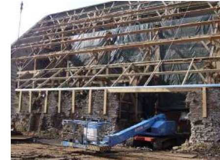
Figure 1.13 New roof construction of the tithe barn for the installation of emergency roofs.
