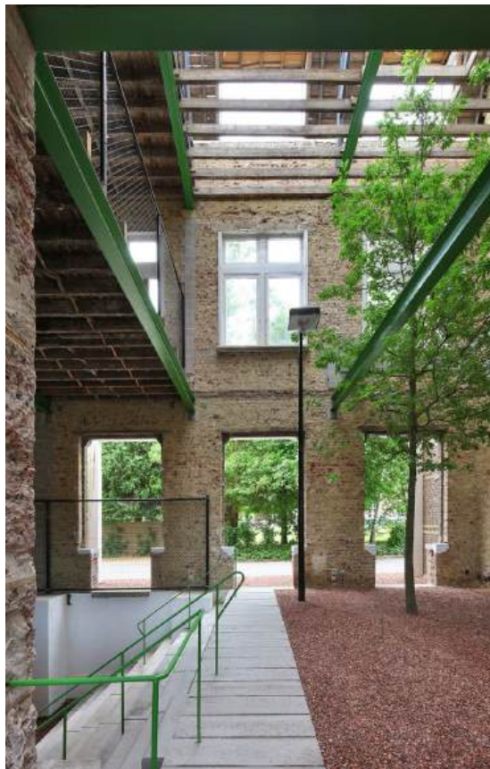
Figure 4.9 Enclosed exterior garden.
