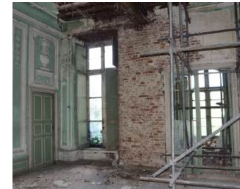
Figure 3.13 Scaffolding supporting the ceiling.
