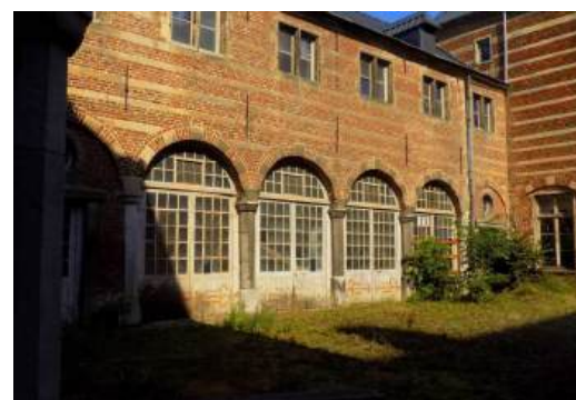
Figure 3.27 West facade fitted with French doors today.
