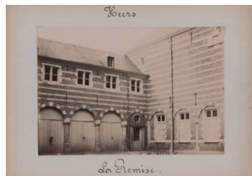
Figure 3.26 Enclosed west facade of the inner courtyard around 1900.
