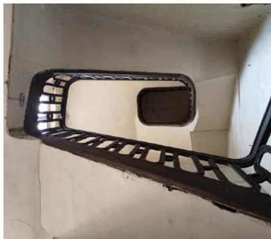
Figure 3.7 Steep, spiral staircase.
