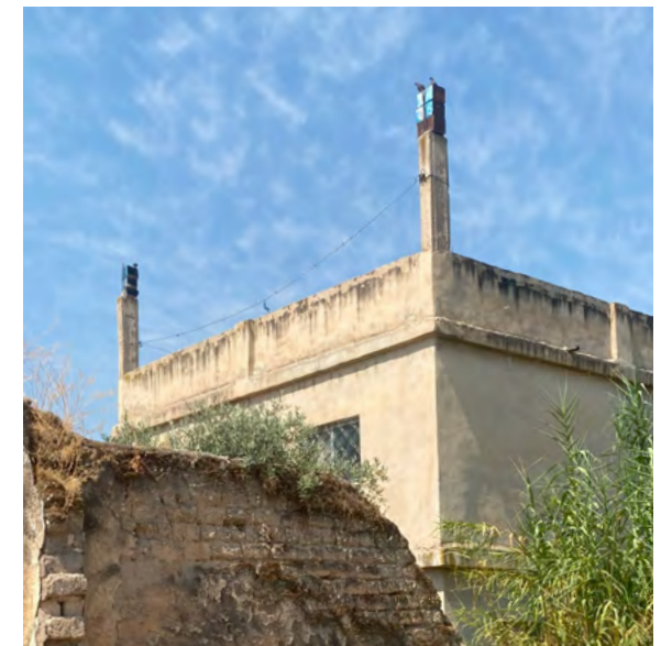
Fig. 12. Extended Columns for Vertical Growth in Al-Zamaliyyah
