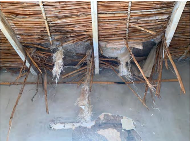
Fig. 29. Broken Mud House Ceiling
