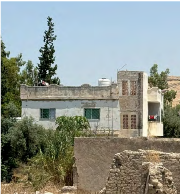
Fig. 38. Reinforced Concrete House with Exaggerated Parapet and Balcony and Claustra Blocks
