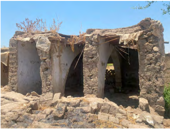
Fig. 33. Structure of Ruined Mud House 3 (R3)
