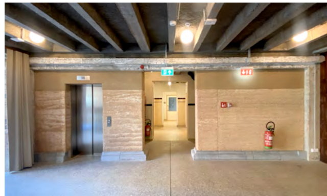
Fig. 8. Hempcrete Wall by BC Architects at USquare Feder
