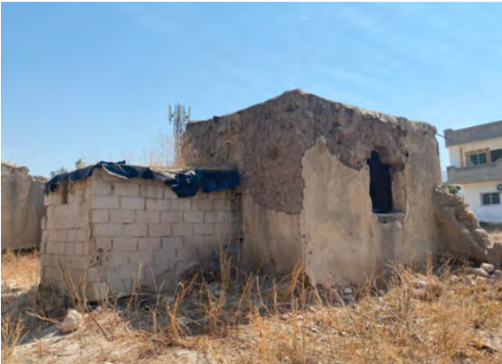
Fig. 36. Vernacular Concrete Block Addition of E1
