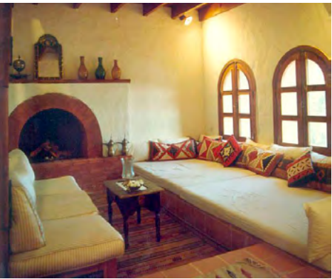
Fig. 43. Mud-Based Built-in Furniture
