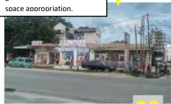
38. A commercial frontage with retail spaces. the interview and observations revealed richness, space generation and interior space appropriation.
