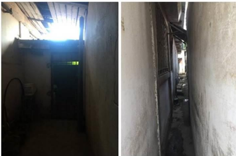
Figure 45: Dark and narrow alleys within a plot along Shekilango Road resulting from piecemeal construction and nonconformity to regulations (source: author, fieldwork 2019).
