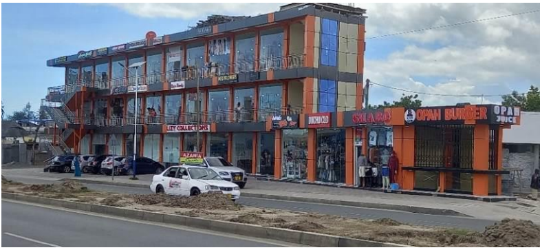
Figure 83: A newly constructed 2-floor commercial building at Sinza Kwa Remmy with commercial spaces on all floors (source: author, fieldwork 2022).
