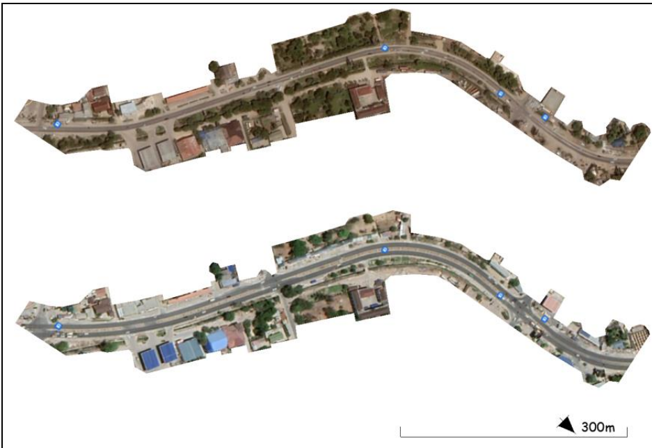
Figure 89: A section of Shekilango Road in 2015 before the road expansion and after the expansion in 2022. 55
