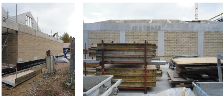
Figure 1. Case 1 - Scharphout, loadbearing and non-loadbearing masonry with CEB (newly built).
