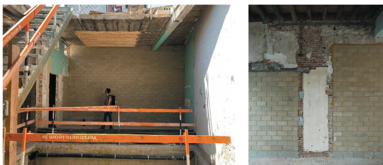
Figure 2. Case 2 - Ostend, non-loadbearing masonry with CEB (renovation).
