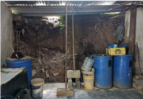
Figure 6: The Community Kitchen collapsed back wall. Soil coming into the space—photo by the author.
