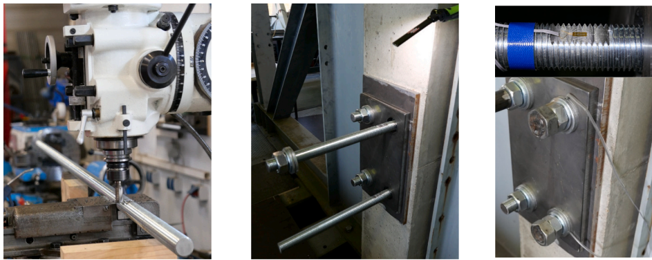
(f) Milling of the threaded rods, insertion into the RC wall, and instrumentation with strain gauges
