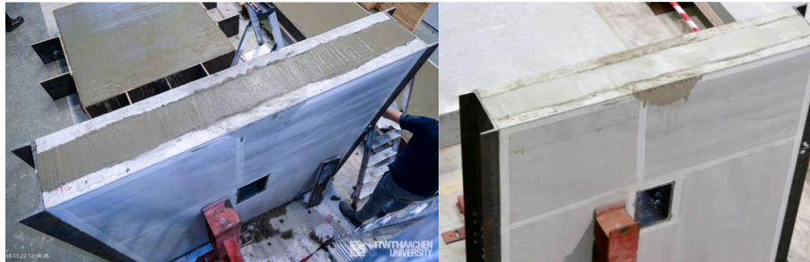
(e) Wall after concrete casting
