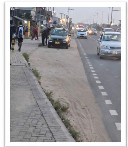
Bus stop without shelter
