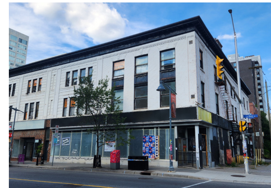
227 Bank Street, Ottawa, Ontario, Canada, built in 1888. Tenants were fully evicted in 2025 in preparation for redevelopment. Image by author.
