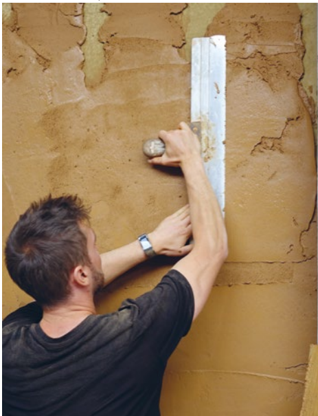
BBB PG hands on explorations: earthen plaster
