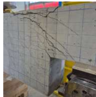
Figure 14. Failure of RE-H
