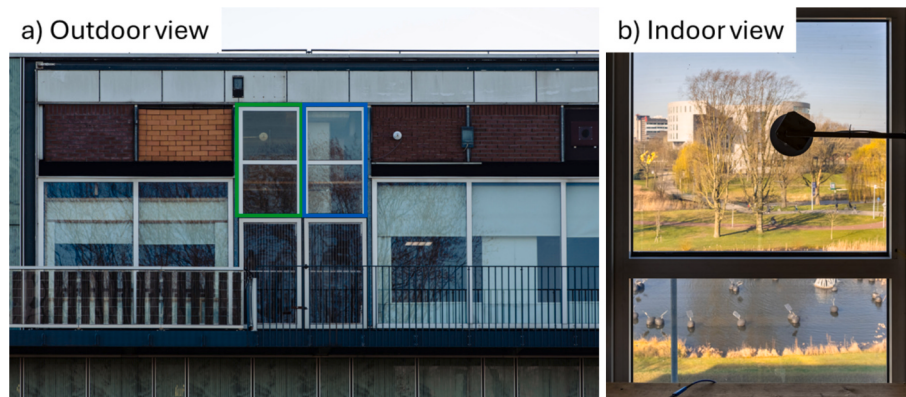
Fig. 2. Window installation at the SolarBEAT test site. a) Westward facing façade with the 2 installed smart windows (green square) and the 2 installed reference IGUs (blue square). b) Look through one of the smart windows from inside out with pyranometer installed at the middle of the window. (For interpretation of the references to colour in this figure legend, the reader is referred to the web version of this article.)
