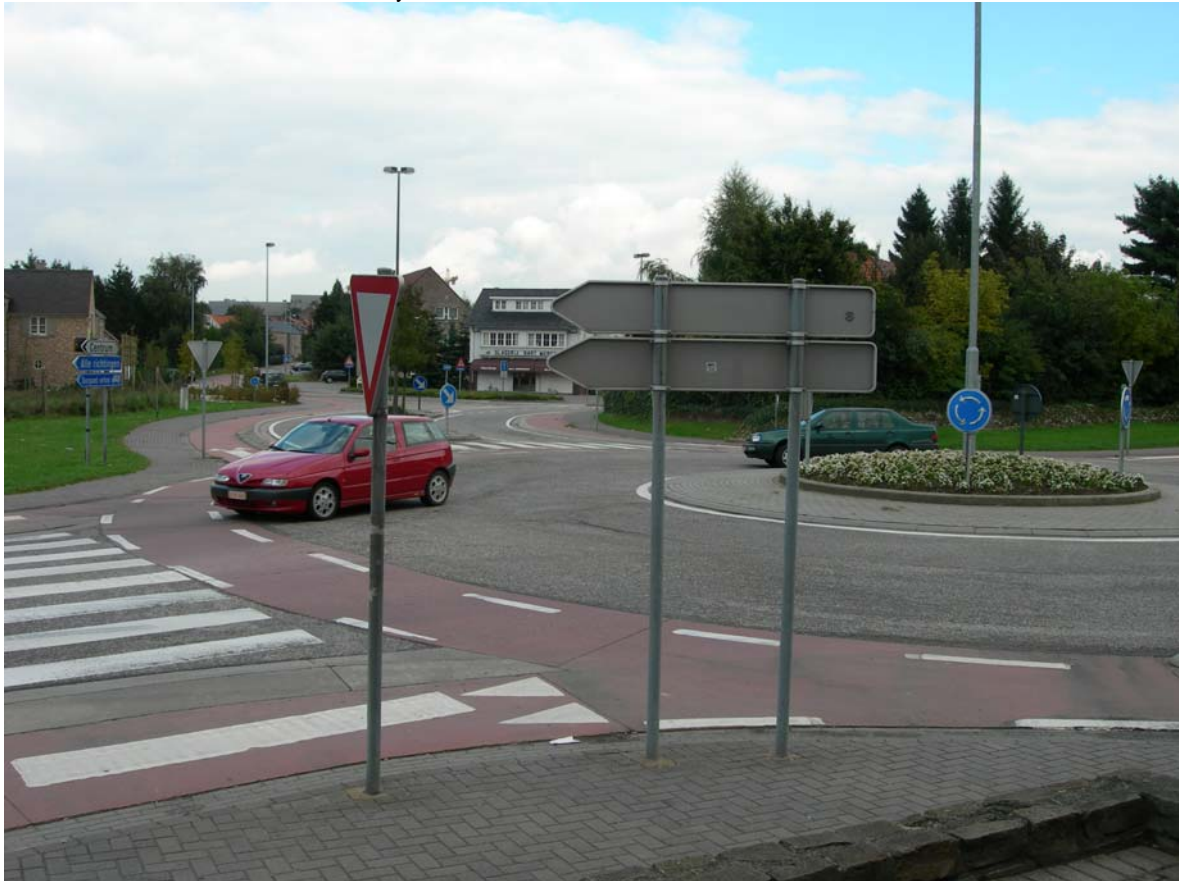
Picture 1 – Roundabout with cycle lanes
